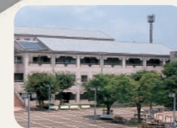
⑤ Laboratory and Training Building
